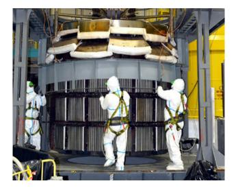
"Unlike VVER-440, VVER-1000 reactors have never been annealed before. Since its walls are thicker, the annealing temperature must be approximately 150°C higher. Why Balakovo NPP Unit 1? Because its reactor vessel is made of steel with higher nickel content," said Vladimir Asmolov, Advisor to Director General of Rosatom.
