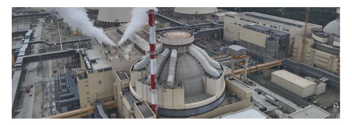
Unit 1 of the Rooppur Nuclear Power Plant has entered one of the most critical pre-commissioning stages as hot functional tests began on the reactor. During the tests, the reactor is gradually heated up, while engineers methodically assess the performance of key components — pumps, pipelines, and heat exchangers — under these conditions. It is essential to monitor how the equipment behaves in operation to make sure it will be safe and reliable once the plant is up and running.
