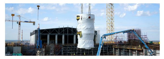
In September, key components for the 300 MW BREST-OD-300 demonstration lead-cooled fast reactor were delivered to the ODEK construction site at the Siberian Chemical Plant. These include a steel casing for the reactor's central cavity, an inner shell for the core basket, and the first of the peripheral cavity casings. There are four such casings in total. All these components were manufactured at the production facilities of Rosatom's Mechanical Engineering Division.
