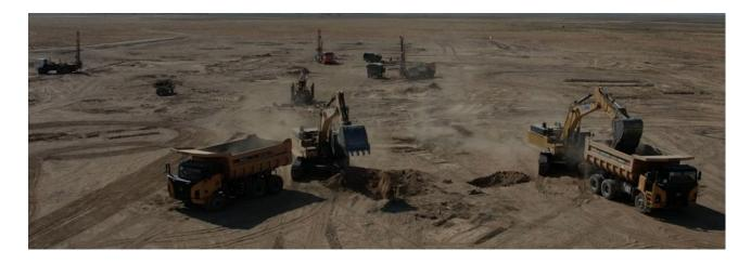
Construction of Uzbekistan's small-capacity nuclear power plant (SNPP) has entered a pivotal phase. It involves excavating a pit for the foundation of a power unit with a RITM-200N reactor to be built in the Farish district of the Jizzakh region to a Russian design. Approximately 1.5 million cubic meters of soil will be excavated for the station, with the pit to reach 13 meters deep.
