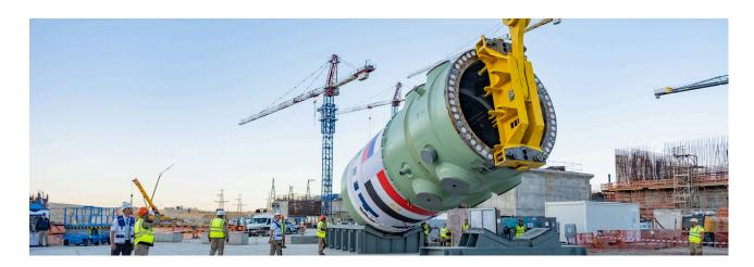
The 340-tonne reactor pressure vessel (RPV) for the power plant's first unit was delivered to Egypt in late October. It passed the incoming inspection before workers proceeded with installation. First, the RPV was lifted from a horizontal to vertical position. Then, workers began lowering it into the reactor pit. All those operations were carried out using a heavy-duty crawler crane with a lifting capacity of 2,200 tonnes.
